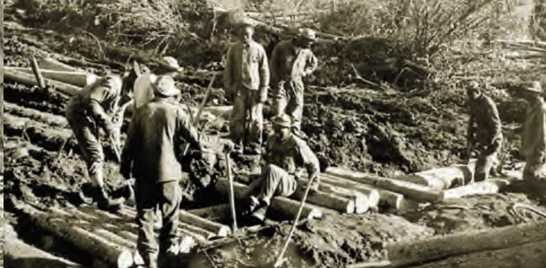
Soldiers constructing a culvert along the Alaska Highway, 1942. (National Archives of Canada Coll., 88/138 #42)
